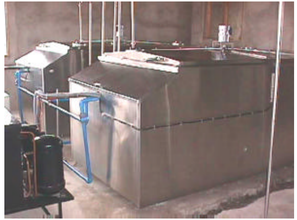
Bulk Milk Coolers – IBT Types 2 x 2000 Ltrs
